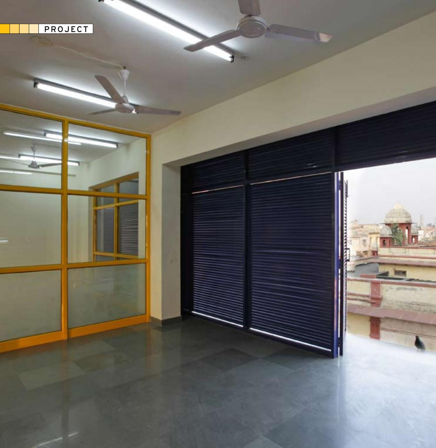
proceed to the first floor for the treatment. This treatment area requires more privacy and has coloured aluminium louvers to provide a visual shield yet allow ample ventilation. A lift designed for carrying stretcher patients has also been installed for emergency treatment.
